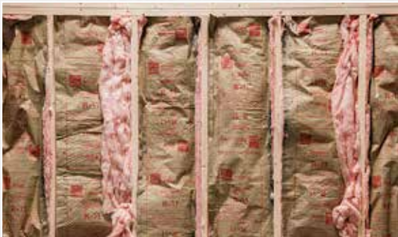
R-13 Batten Insulation In Walls & Ceiling
