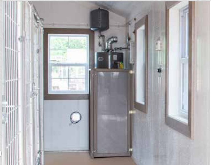
Radiant Floor Heat System
