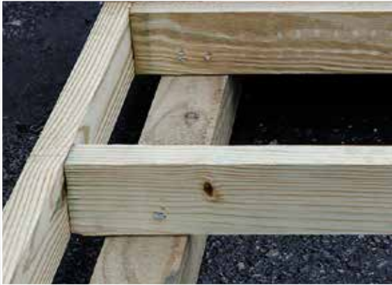
Pressure Treated 2x4 Floor Joists 4x6 Runners
