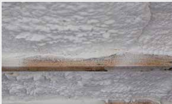
R-13 Closed Cell Spray Foam Insulation in Floor
